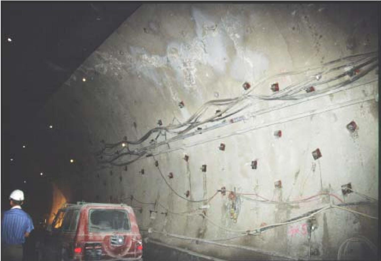
Figure 8. Damage to the tunnel lining due to the anisotropic deformations between stations 1785 and 1800.
