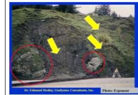
**Situation D** illustrates the common condition of variations in the block proportion within the rock mass. Failures can be expected through those regions where there is continuity within a low-proportion, weaker domain.
