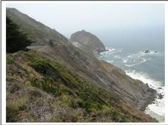
The Devil's Slide, on the abandoned section of Highway 1 here, has a long, very pricey history, having destroyed previous roads and a railway since the 1890's. Failure occurs as kinematically unstable blocks of steeply dipping, faulted and sheared rocks which daylight on the very steep slopes continually destabilized by the ocean. The twin-bore 4100 feet long by-pass tunnel was constructed, with difficulty, between 2005 and 2011.
